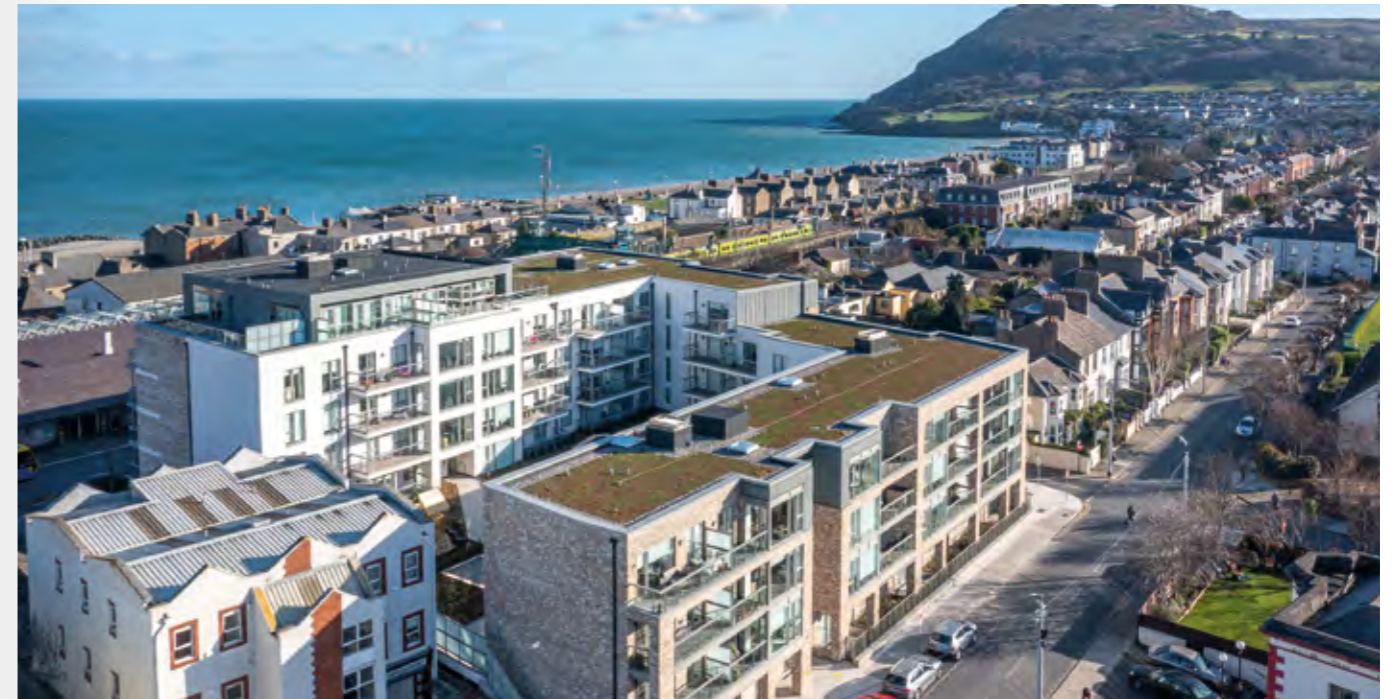
Apartment Development at Bray, Co. Wicklow developed by Glenveagh and purchased by Ardstone
