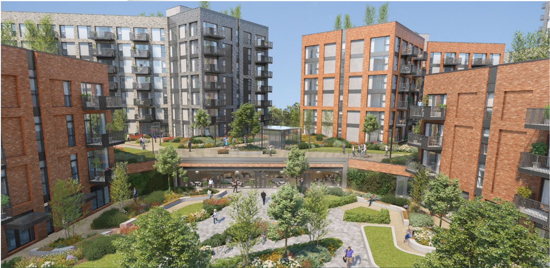
8th Lock, Royal Canal Park, Dublin 15 being developed by Ballymore & forward funded in a €200 million transaction with Union Investment in H1 2021
